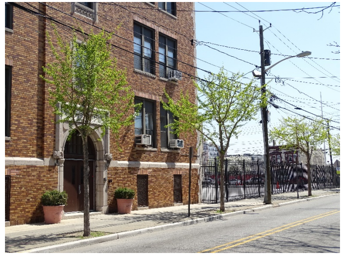
Newly planted Ginkgo trees that will become entangled in overhead wires as they grow.
